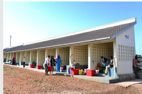
The Isiolo Livestock Market, constructed under REGAL-AG
