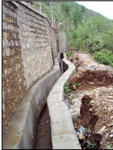
Figure 1: Irrigation Canal Cleared Through ACDI/VOCA CAP Project
